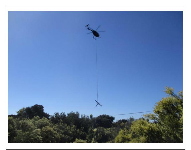
**Photo 4:** Crews were observed cutting off old wooden poles above communications lines and removing pole tops via helicopter external loads along C 449 (P45925, above).
