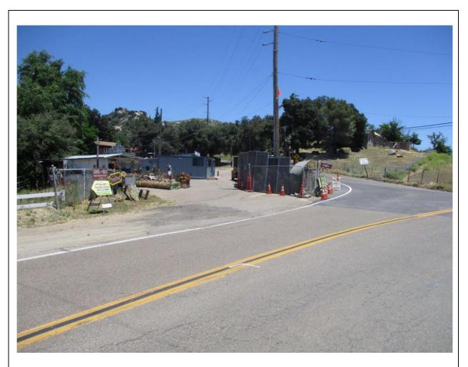
**Photo 3:** Noise barriers were observed being implemented at Z173060 (TL 629A) during micropile drilling activities to reduce noise in accordance with MM NOI-1.
