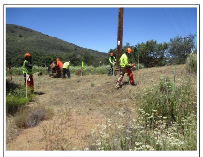
**Photo 1:** A crew was observed clearing vegetation within the approved workspace at Z173101 (TL 629A) in accordance with MM BIO-1. A biological monitor was present on site in accordance with MM BIO-03, and a set of fire tools was placed within 50 feet of activities in accordance with the CFPPP fire prevention matrix (off CNF land - FPI Normal).
