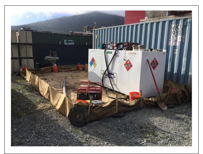
**Photo 6:** Containment placed under the generator and fuel tank at the Merrigan Staging Yard (TL 629A) in accordance with the SRNP and MM PHS-2.
