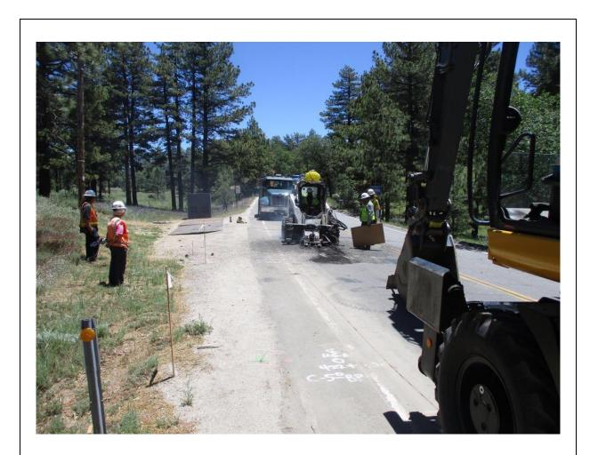
**Photo 5:** During asphalt grinding at Station 422+74 (C 440) in preparation for vault excavation and steel plate installation, water was applied at the recommendation of the SDG&E fire coordinator for fire risk mitigation in accordance with the fire prevention matrix in the CFPPP. Cultural resource monitors were present on-site for upcoming vault excavation work in accordance with the HPMP, MM CUL-1, and APM CUL-04.
